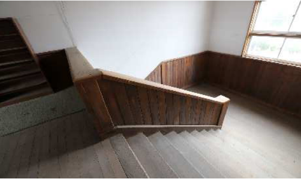
階段腰壁手摺
